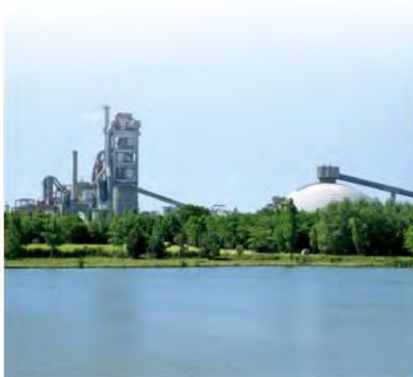
Usine Lafarge – Saint-Pierre-la-Cour
